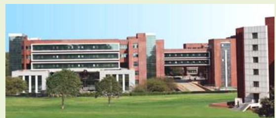
Connectors between buildings to reduce energy consumption
