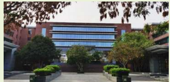
Glass façade for Daylight utilization
